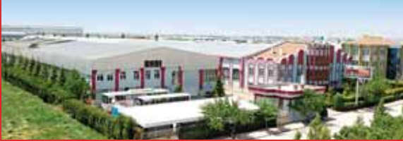
Piston & Piston Pin Production Facility Piston & Pim Fabrikası
