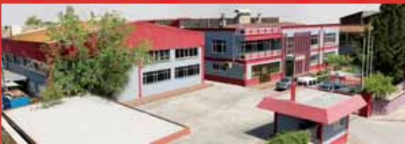
Cylinder Liner Production Facility Motor G mleđi Fabrikası
